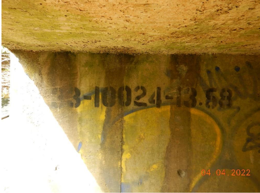
BRIDGE NUMBER - BARREL #1 - EXTERIOR WALL RIGHT
